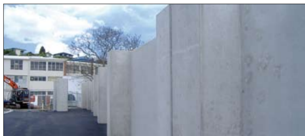
BUILT TO LAST: This bund wall is 3 metres high.
