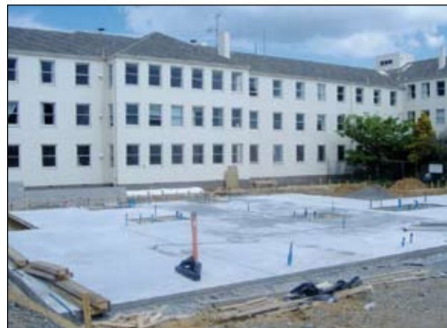
INPATIENT CENTRE: Concreting was completed in November.
