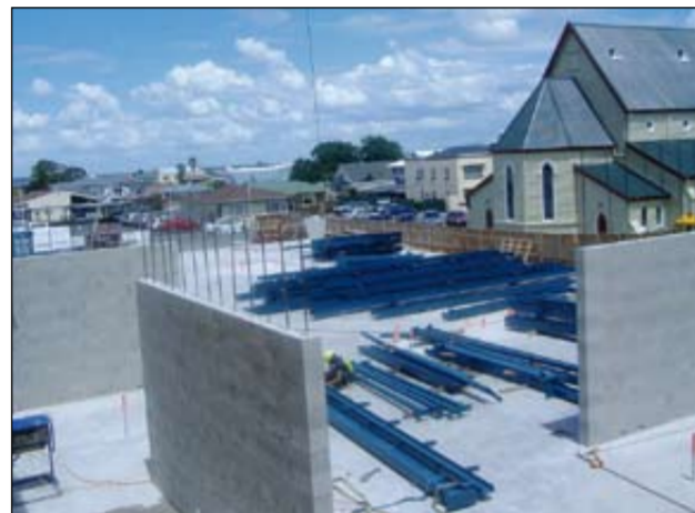
CLINICAL CENTRE: Foundations were laid in November.
