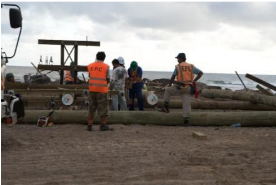
Rebuilding already happening. Power lines going back up rapidly
