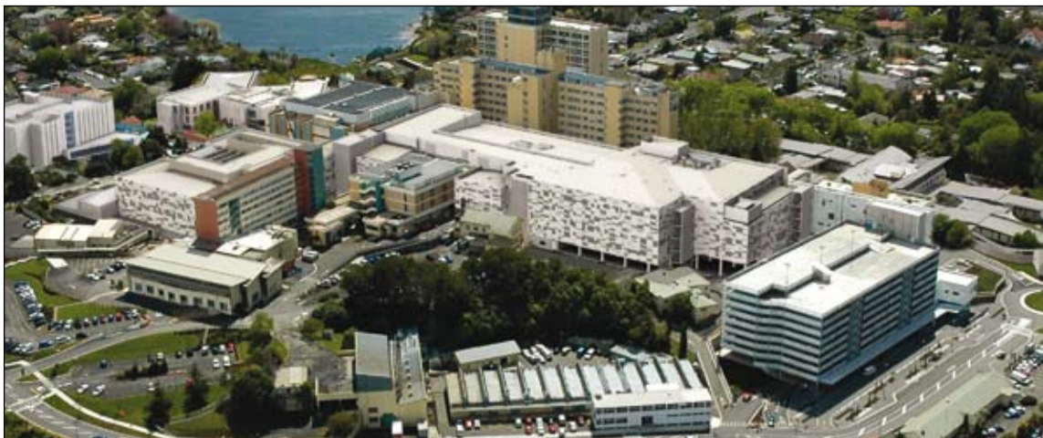
BIG BUILDING: When built, Waikato Clinical Centre will link into the new carpark building, improving access into the hospital.
